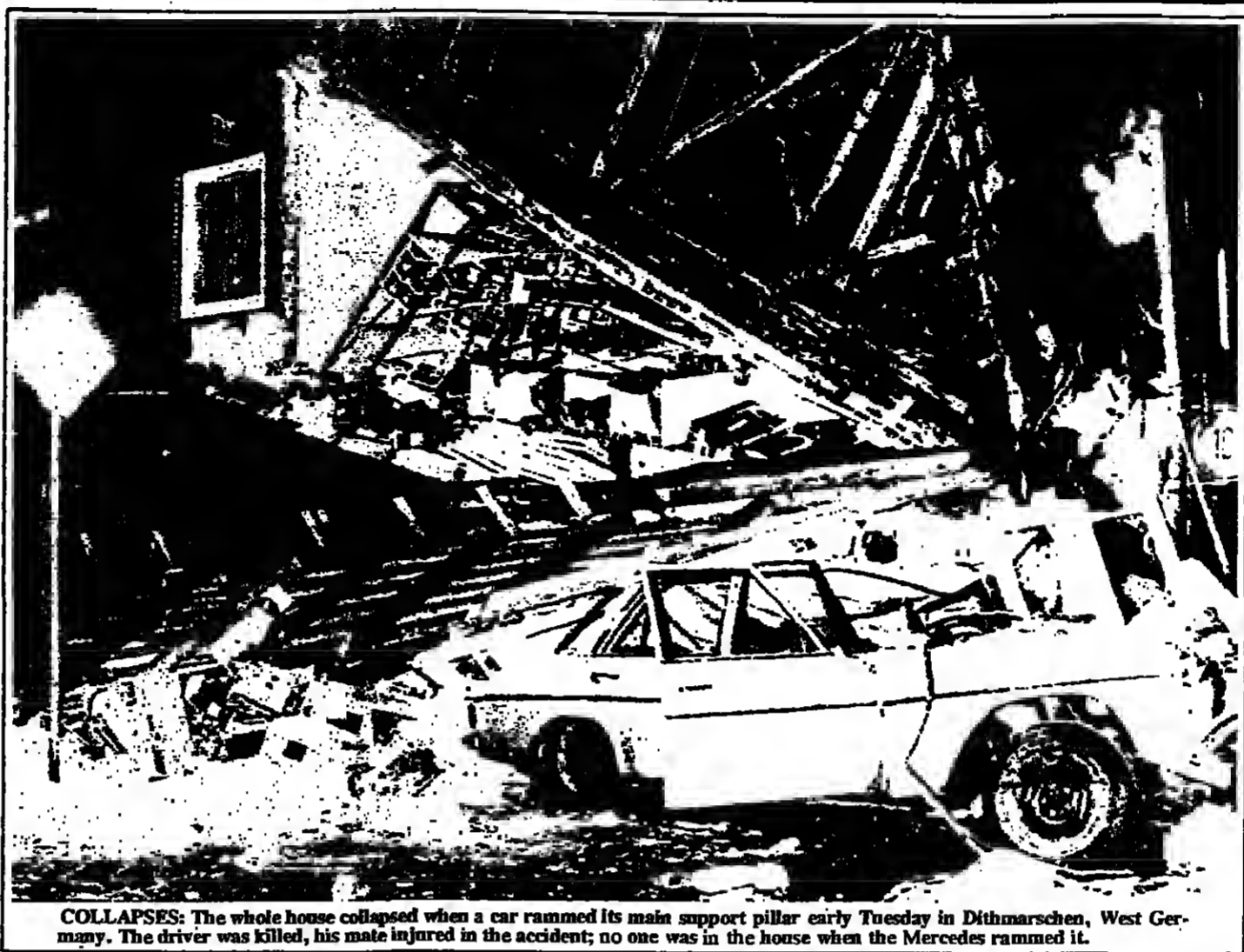
COLLAPSES: The whole house collapsed when a car rammed its main support pillar early Tuesday in Dithmarschen, West Germany. The driver was killed, his mate injured in the accident; no one was in the house when the Mercedes rammed it.
